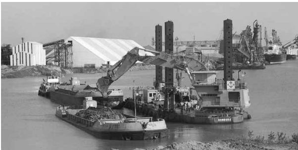
Figure 2: Dredger in operation with two barges and a tug. The landing manoeuvre of the barges requires experienced captains in order to keep the disruption of digger usage short.
