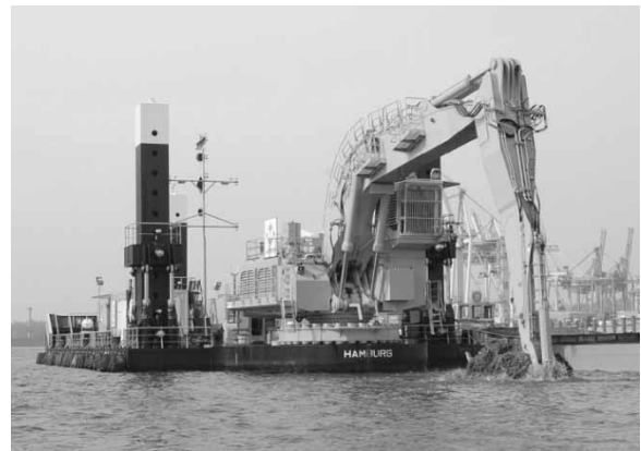
Figure 1: A dredging platform with a bucket excavator, bucket size 14m 3 .
