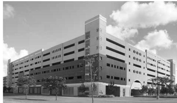
Figure 1: A parking garage with approx. 2,000 parking spaces on six levels.
