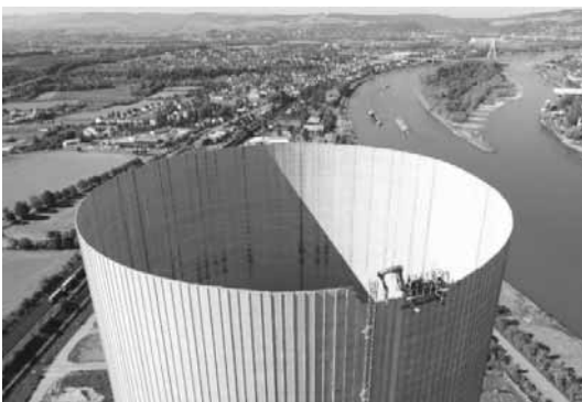
Figure 1: Demolition of the cooling tower in Mühlheim-Kährlich with the demolition excavator.
