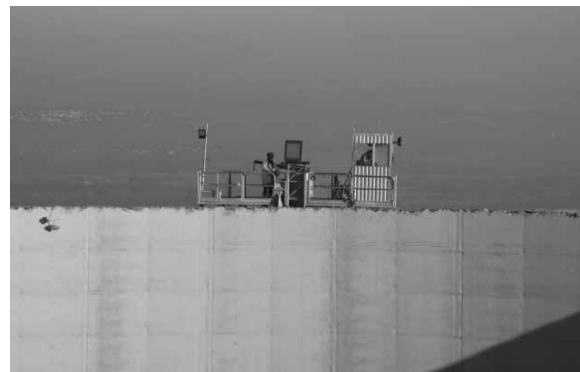
Figure 2: Conventional operation of the excavator with a handheld remote control from a platform on top of the cooling tower.
